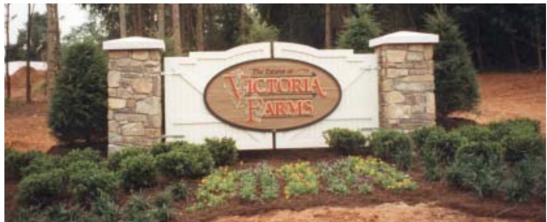
Letters are two layers of Sintra [Alcan Composites USA, Inc., 800-626-3365, www.alcancomposites.com ] cutouts finished with Matthews two-part polyurethane [Matthews Paint Co., 800-323-6593, www.signpaint.com ], on 4-by-6-ft. sandblasted cedar panel finished with acrylic latex paints. The gate is grooved plywood framed with cedar, finished with acrylic paints, mounted on stone piers.
