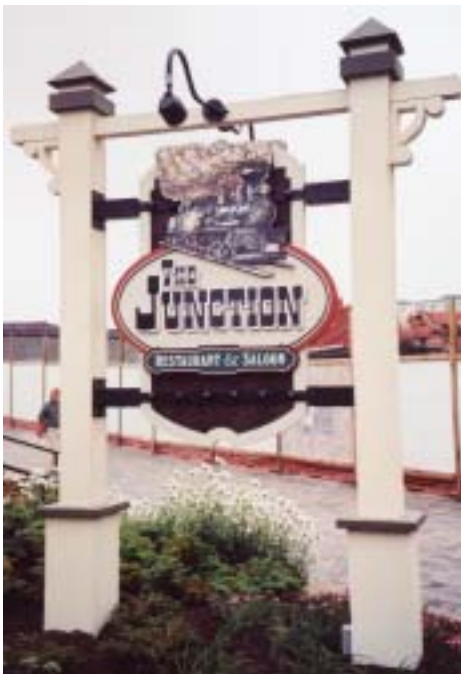
Main copy is sandblasted in Sign-Foam high-density urethane board panel. Train graphic is vinyl, printed on the Gerber Edge®, mounted on 1/4-in. PVC panel. Restaurant & Saloon is vinyl, mounted on 1/2-in. PVC panel. All are mounted on sandblasted cedar panel, held by iron supports to cedar posts and cross arm. Overall size is 8 by 9 ft.
