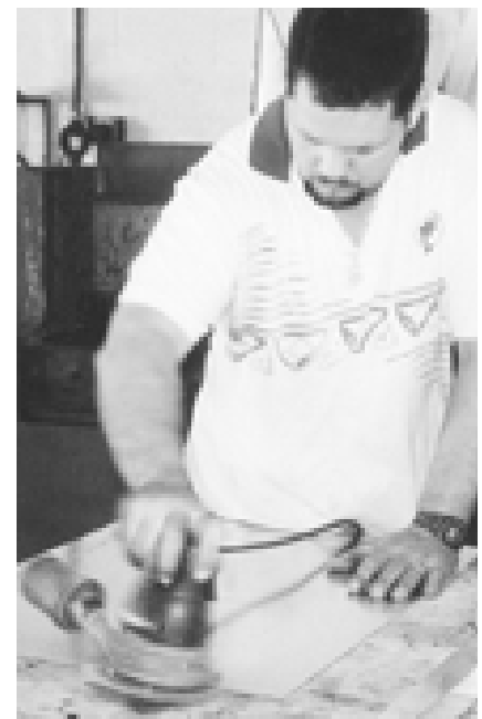
Sanding the panel
