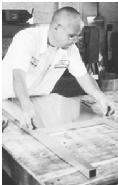
Fitting the panel
