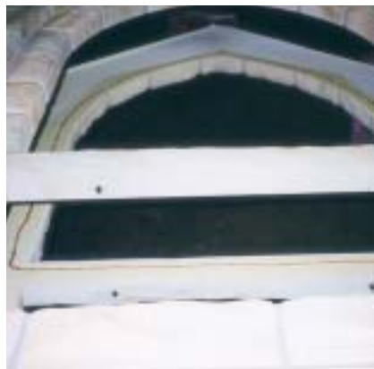
Figure 29. Applying the glue to the body before inserting panels
