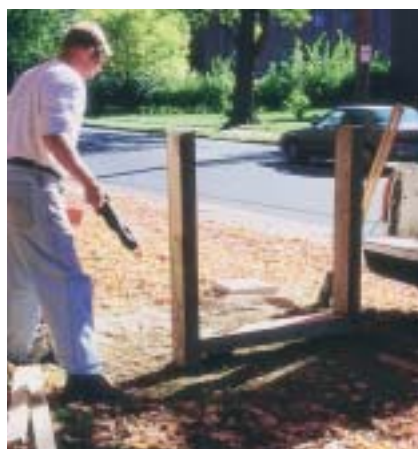
Figure 34. My brother, Greg, installs the posts.
