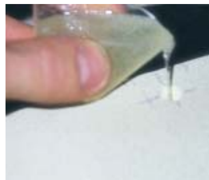
Figure 28. Pouring epoxy into the oversized hole where the screw will be inserted
