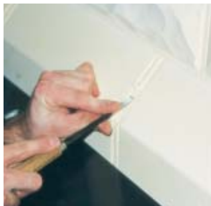
Figure 12. Some of the mortar joints on the angled pieces had to be carved by hand.
