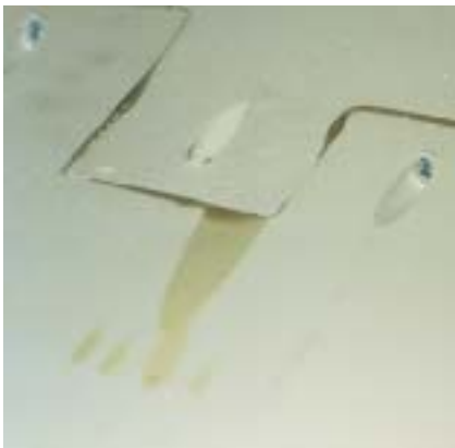
Figure 4. The two sections were joined using urethane glue and galvanized sheetrock screws.
