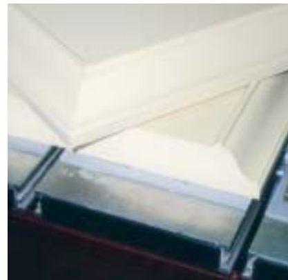
Figure 15. The routed caps with the look of crown molding
