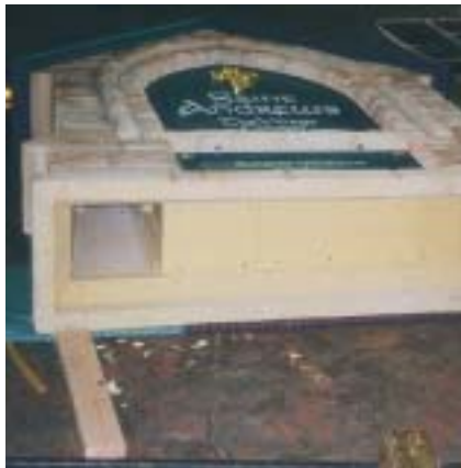
Figure 33. The base was screwed and glued in place. Note the holes are where the posts slide up through.
