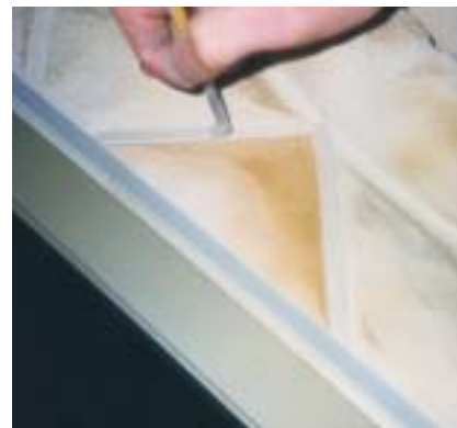
Figure 26. Painting the mortar with a fitch
