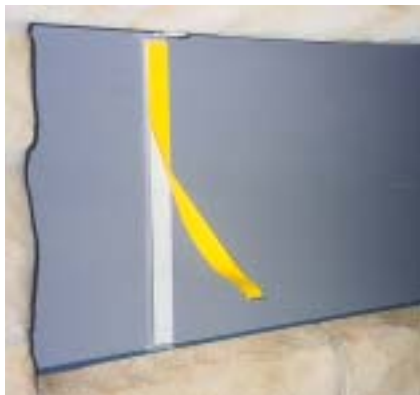
Figure 31. Double-sided tape aided in alignment of the brackets.
