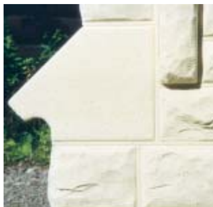
Figure 14. Slight sandblasting on the HDU gives a texture similar to real stone.
