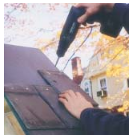
Figure 35. Screwing the slate onto the roof
