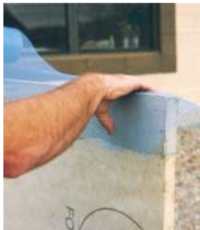
Figure 6. Backwrapping an edge
