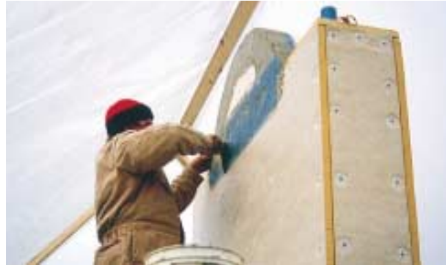
Figure 8. Applying base coat to seams and corners
