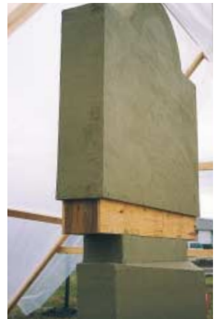
Figure 10. Base coat is dry and ready for finish coat.
