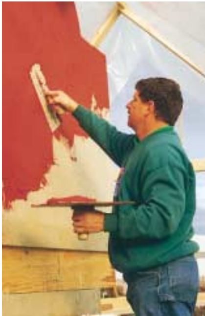
Figure 11. Applying finish coat with metal trowel
