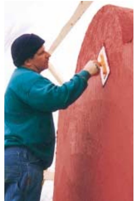
Figure 12. Finish troweling with plastic trowel
