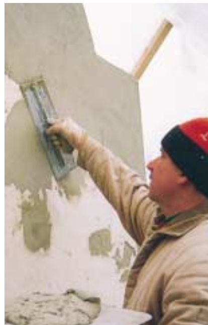
Figure 9. Applying base coat to entire sign
