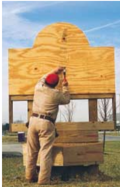
Figure 4. Skinning with plywood
