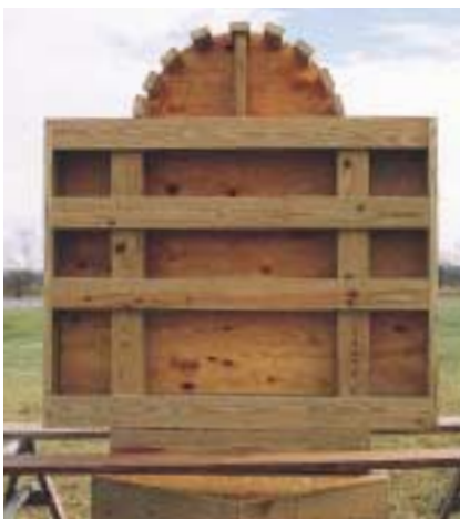
Figure 5. Note bracing for top arch
