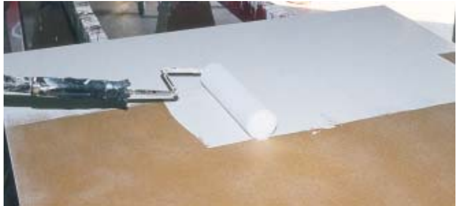
Figure 15. The 9-in. foam roller cover is saturated with paint. I apply a heavy layer of primer, so the roller goes through the paint several times and then is paletted over the ribbed portion of the tray.
