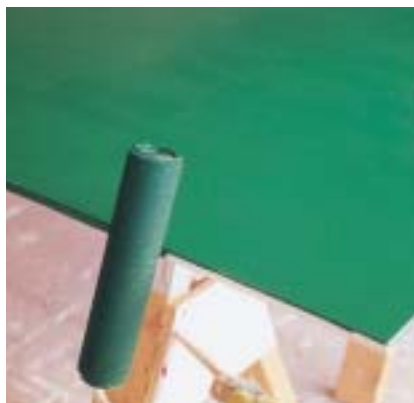
Figure 23. The edges always receive special attention. Notice the bubbles in the paint.
