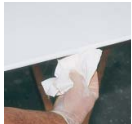
Figure 18. A foam brush is used to smooth out the drips that have run under the panel, or sometimes just a swipe with a paper towel cleans up the mess.
