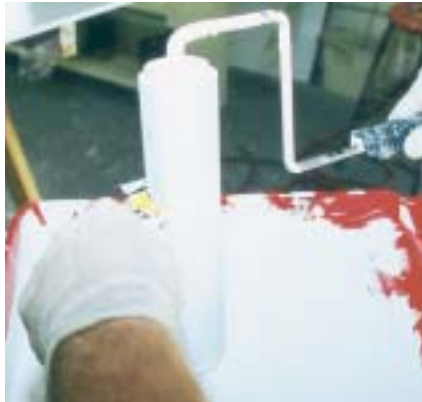
Figure 19. To clean the excess paint out of the roller I use a paint scraper that has a circular notch in the side. The leftover primer is pushed down into the tray. Excess paint is cleaned out of the tray by using the foam brush, then put back into the can. The paint lid is secured with a rubber mallet.
