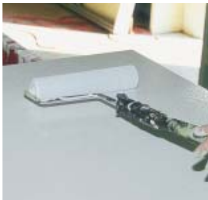
Figure 16. After the panel is covered the primer is rolled in vertical columns at a 90-degree angle to the first passes. This further smooths out the paint and reduces the ridges built up by the edge of the foam cover.
