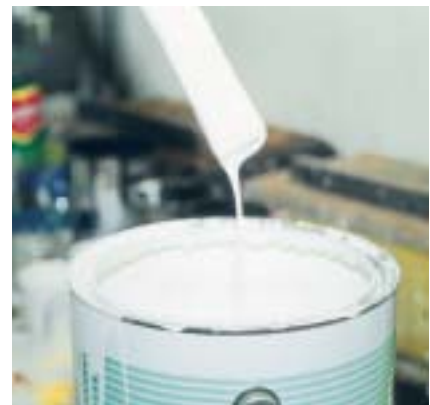
Figure 13. The primer is stirred and the concoction is fine-tuned until it runs off the stick at just the right consistency. Don't ask me what that is—it just looks right. Kind of like buttermilk, more or less.
