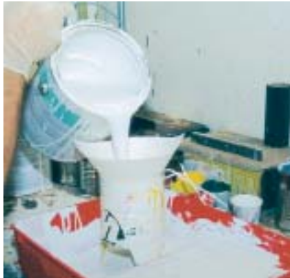
Figure 14. The primer is poured through a strainer into a paint tray. The high tech contraption that holds the strainer is a coffee can with the bottom cut out. The attached wire is for hanging it over the side of a trash can when not in use.
