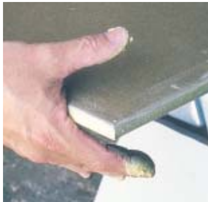
Figure 7. The palm is the perfect form for shaping and smoothing the putty. This is done every few feet before the putty hardens.
