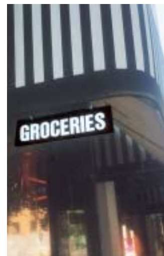
Signs hanging from awnings can be very noticeable. (Check the code for minimum height above ground level.)
