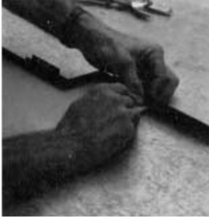
Figure 7. When you need to make an outside bend, use a metal scribe to scratch the trim where you need to notch it. Taking a little extra care to mark the bends accurately is well worth it. You'll get a neater job, plus save time and material, too.
