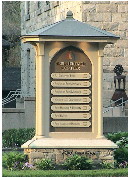
Hand-carved incised gilded lettering on 4-by-9-ft. high-density urethane board structure. The bronze letters are mounted on standoffs on a stone base. "It was great to have full reign over concept, design and fabrication," says Shane. "We designed the bases, which were built to our specs by a contractor affiliated with the site. We also subcontracted the copper cladding on the roof."
