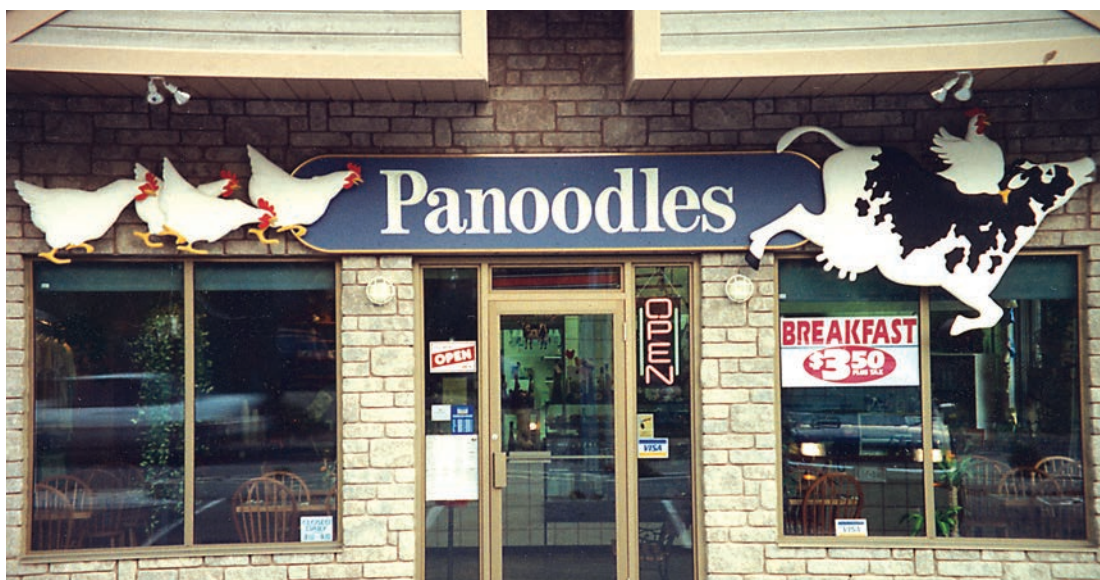
Hand-carved incised lettering on 4-by-23-ft. high-density urethane board with a gilded cove. The cow and chickens are shaped from 2-in. high-density urethane board mounted on standoffs.
