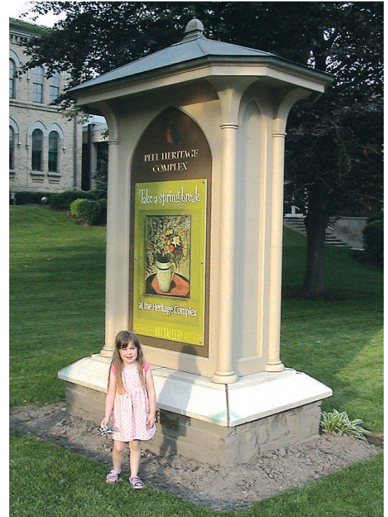
Hand-carved incised gilded lettering on 5-by-12-ft. high-density urethane board structure. The bronze letters are mounted on standoffs on a stone base. "This project was too large to assemble in our studio," says Shane, "so we drew it to actual size on the computer, fabricated it to computer measurements and assembled it on site."
