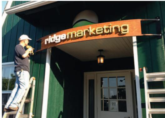
**5. Assemble and install: 3 hours** The logo was installed using a french cleat so that there were no visible fasteners, then the sign was bolted to the wall.
