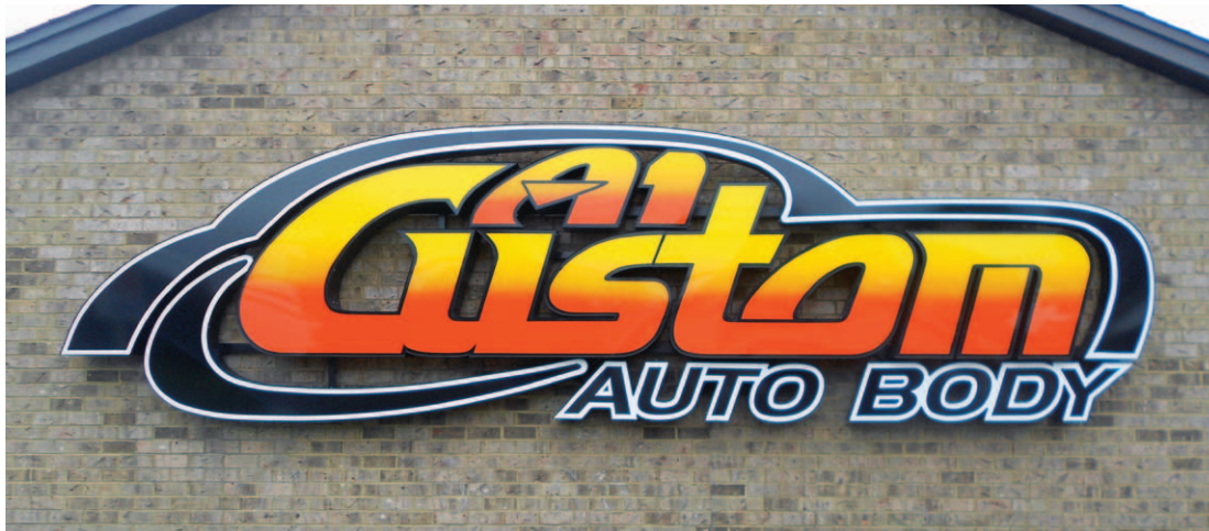
Acrylic faces on custom aluminum cabinets, with LED lighting; 6-by-20-ft. overall. "This was fabricated and installed by Neolite Signs, which was my son Michael's former company," says Mike. "Jay designed the logo and did the paint work."
